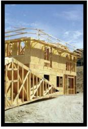
Roof line fall protection has been installed, and is providing an OSHA acknowledged system for workers to safely and efficiently complete all work at and above the roof line. Once The WHALEN-JACK system is installed it will eliminate the workers need to be in fall arrest systems.
