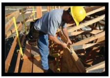
Eave blocking is at an ergonomically favorable height and is safely and easily installed. All necessary roof hardware can be installed.
