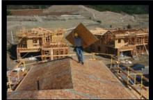
The WHALEN-JACK system is providing a complete fall protection system at the exterior of the building allowing workers to complete sheeting, gutters and roofing safely and efficiently without the use of lanyards or other fall arrest systems.
