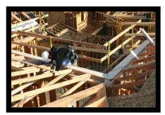
Eave sheeting is at an ergonomically favorable height and is safely and easily installed.
