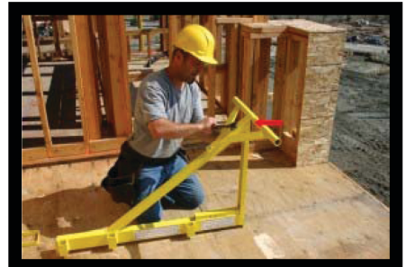
4. Tighten bolts with cross member in correct position.
