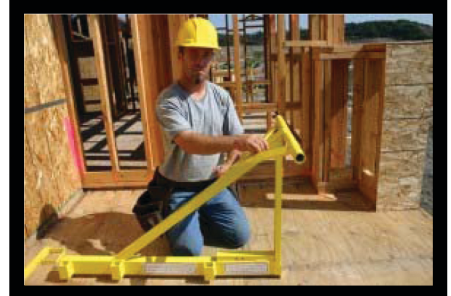
1b. Place triangle cross member support on diagonal of mainframe (orient cross members as shown in picture) .
