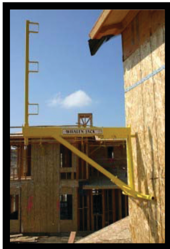
5. Assembly of The WHALEN-JACK is complete.
