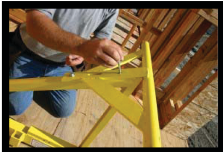
2. Place washer and nylon insert lock nut on bolts.
