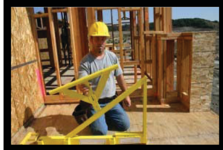
1a. Place triangle cross member support on diagonal of mainframe (orient cross members as shown in picture) .
