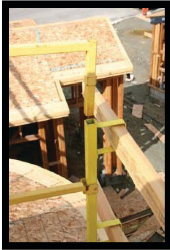
Slide End Gate into handrail and pin in place.
